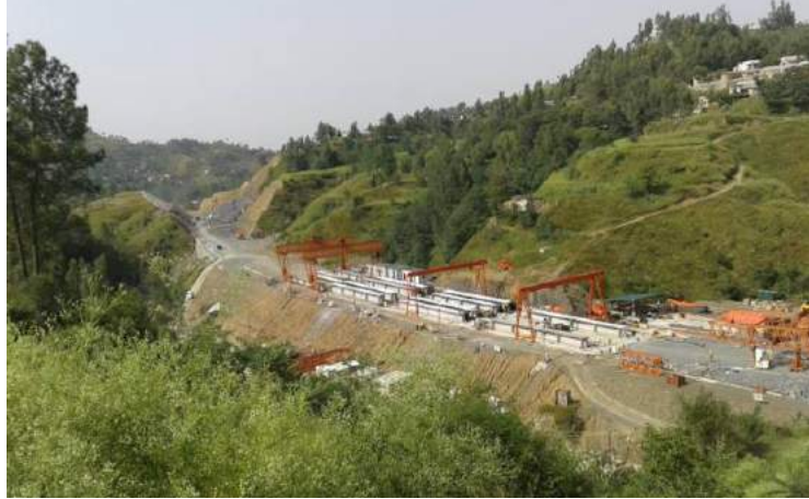
Figure 5 KKH Phase-II (Thakot-Havelian Section)
